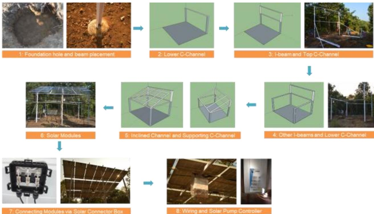
Figure 18: Pictorial representation of installation of SPIS
